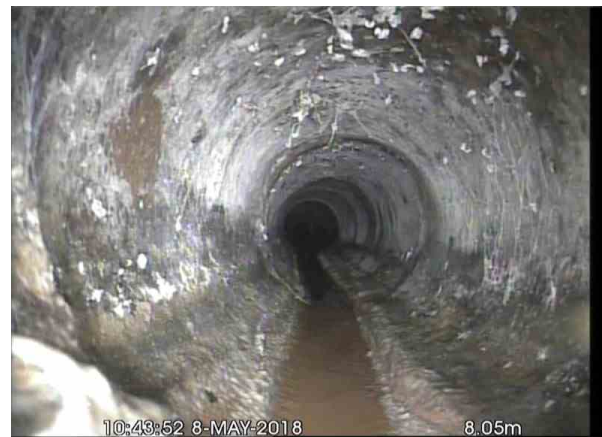
, 00:00:49, 8.05 m Material changes to vitrified clay
