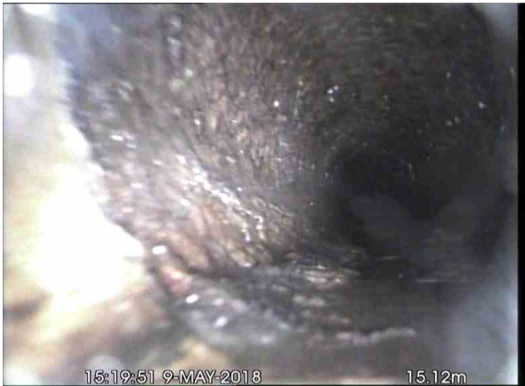
, 00:01:38, 15.12 m Material changes to cast iron
