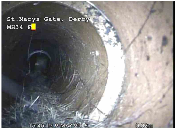
, 00:00:02, 0.02 m Roots, mass, 5% cross-sectional area loss, start
