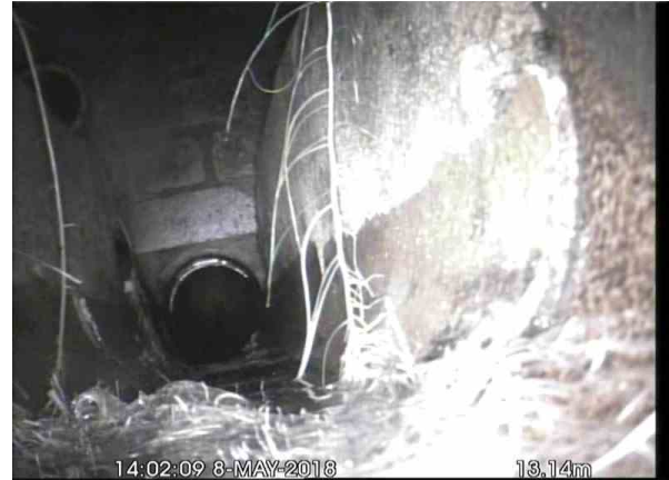
, 00:01:28, 13.14 m Finish node type, manhole, reference number: MH14 X
