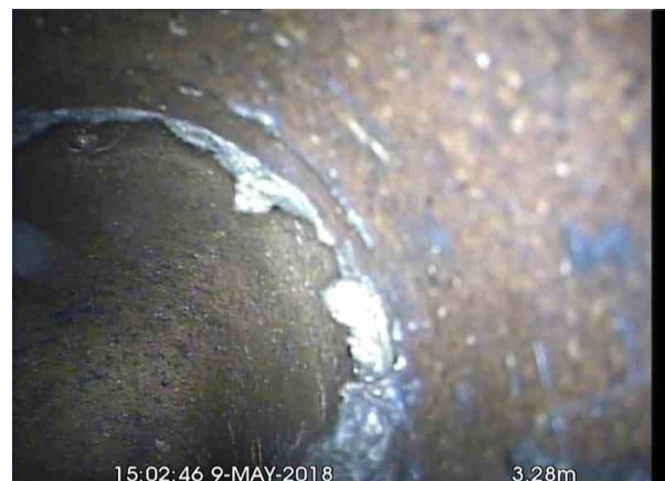
, 00:00:31, 3.28 m Finish node type, gully, reference number: Gully
