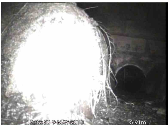
, 00:00:32, 5.91 m Finish node type, manhole, reference number: MH17 X
