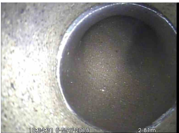
, 00:00:29, 2.81 m Finish node type, other special chamber, reference number: Downpipe, Internal
