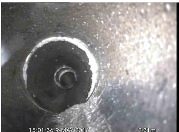
, 00:00:22, 2.31 m Roots, mass, 5% cross-sectional area loss, finish
