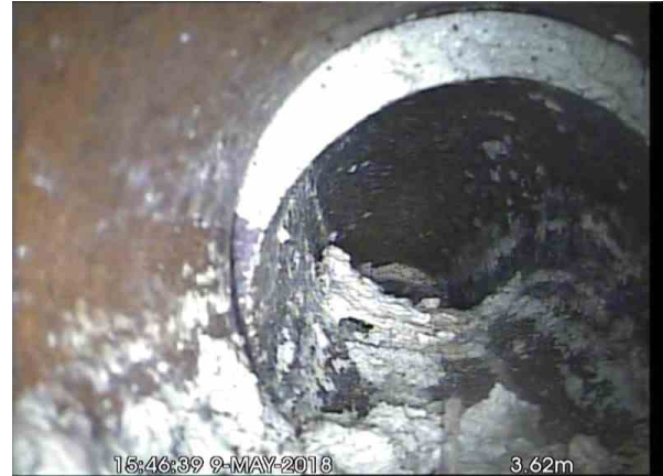
, 00:00:20, 3.62 m Survey abandoned, Unable to pass displaced joint
