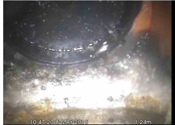
, 00:00:19, 1.24 m Finish node type, gully, reference number: Gully
