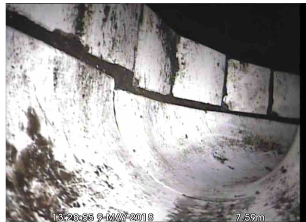
, 00:01:18, 7.59 m Finish node type, manhole, reference number: MH22 B
