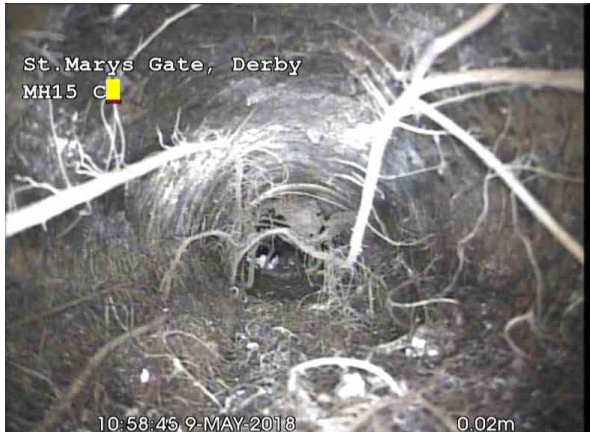
, 00:00:01, 0.02 m Roots, mass, 15% cross-sectional area loss, start
