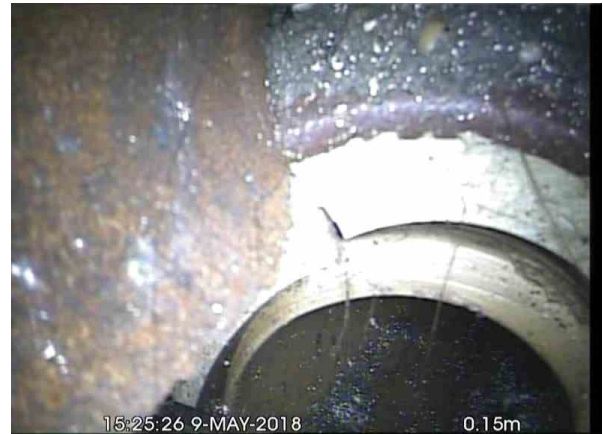
, 00:00:00, 0.15 m Survey abandoned, Unable to pass displaced joint
