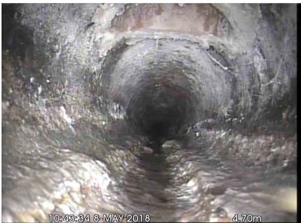
, 00:00:31, 4.70 m Connection other than junction at 12 o'clock, diameter: 100mm
