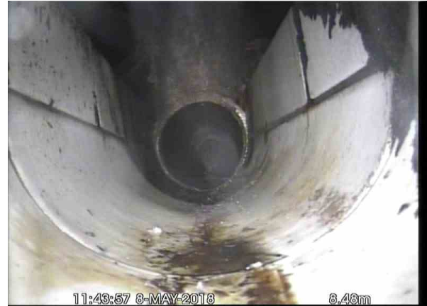
, 00:01:13, 8.48 m Finish node type, manhole, reference number: MH8 X
