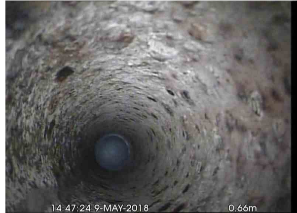
, 00:00:27, 0.66 m Finish node type, other special chamber, reference number: Downpipe, Internal
