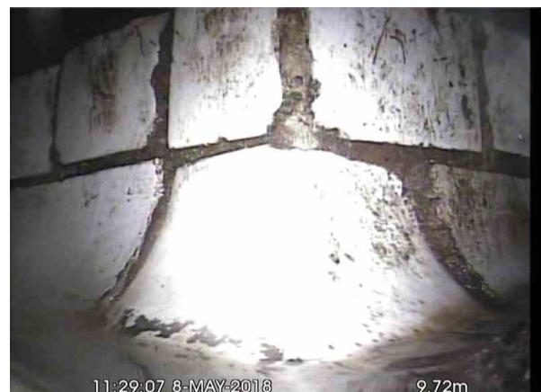
, 00:01:23, 9.72 m Finish node type, manhole, reference number: MH7 X
