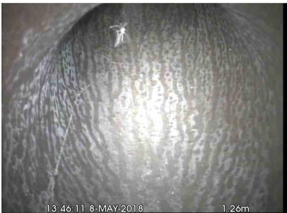
, 00:00:20, 1.26 m Finish node type, other special chamber, reference number: Downpipe, Internal
