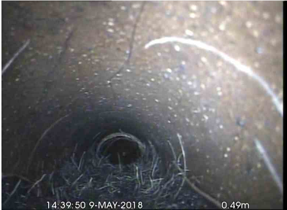
, 00:00:07, 0.49 m Roots, mass, 10% cross-sectional area loss, start
