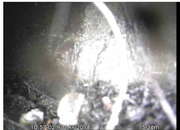
, 00:01:25, 15.36 m Finish node type, manhole, reference number: MH16 X
