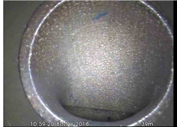
, 00:00:22, 1.39 m Finish node type, gully, reference number: Gully
