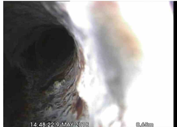
, 00:00:16, 0.68 m Finish node type, other special chamber, reference number: Downpipe, Internal
