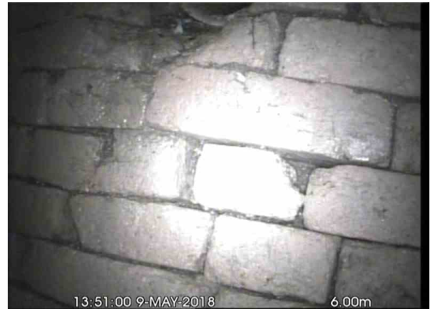
, 00:00:42, 6.00 m Finish node type, manhole, reference number: Main Sewer
