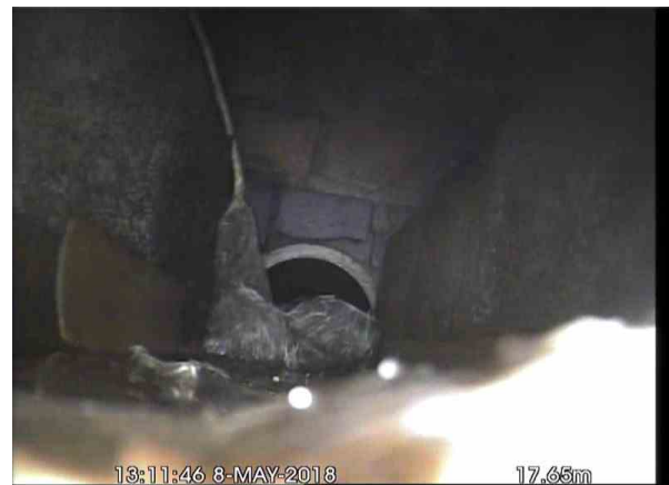
, 00:01:33, 17.65 m Finish node type, manhole, reference number: MH13 X
