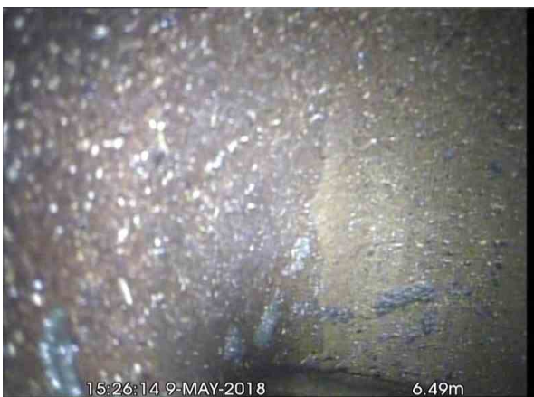
, 00:00:29, 6.49 m Finish node type, gully, reference number: Gully
