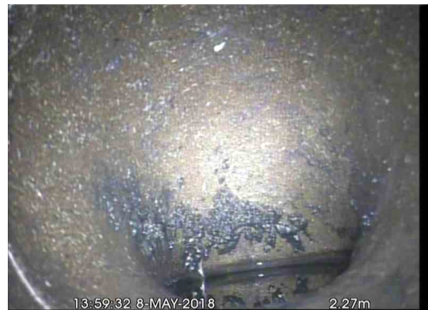
, 00:00:21, 2.27 m Finish node type, gully, reference number: Gully
