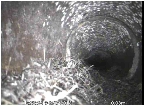
, 00:00:06, 0.08 m Roots, mass, 10% cross-sectional area loss, start
