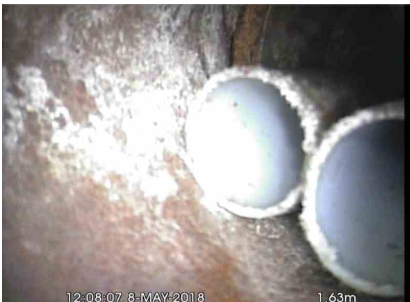
, 00:00:25, 1.63 m Survey abandoned, Unable to pass obstacle
