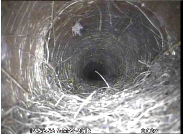
, 00:00:04, 0.02 m Roots, mass, 15% cross-sectional area loss, start
