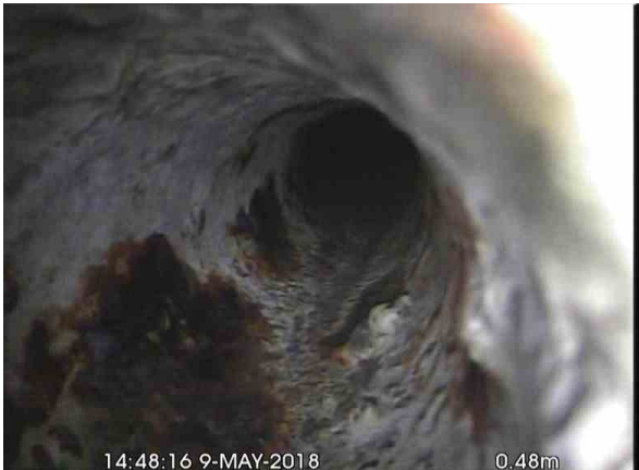
, 00:00:10, 0.48 m Material changes to cast iron
