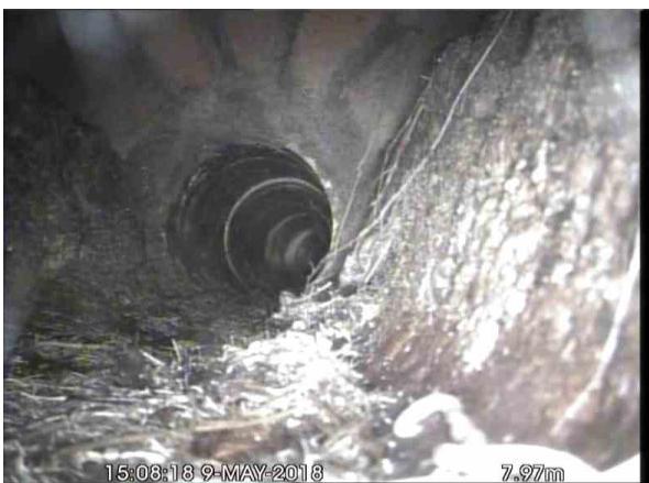
, 00:00:43, 7.97 m Finish node type, manhole, reference number: MH30 X
