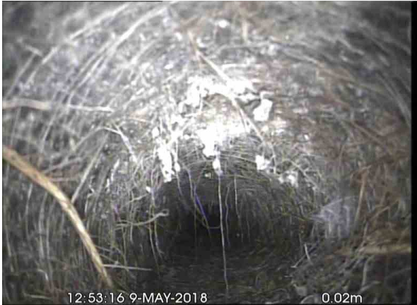
, 00:00:09, 0.02 m Roots, mass, 15% cross-sectional area loss, start
