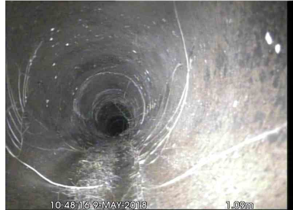
, 00:00:13, 1.09 m Roots, mass, 5% cross-sectional area loss, start
