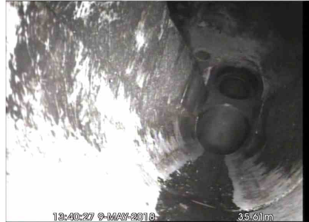
, 00:05:13, 35.61 m Finish node type, manhole, reference number: MH23 B
