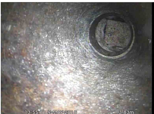
, 00:00:32, 3.83 m Finish node type, other special chamber, reference number: Capped
