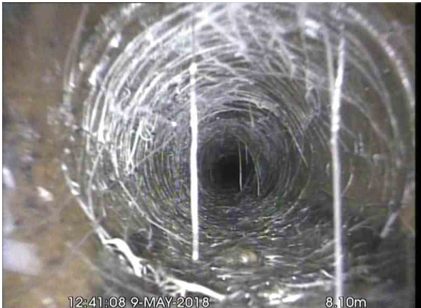
, 00:00:55, 8.10 m Roots, mass, 5% cross-sectional area loss, start
