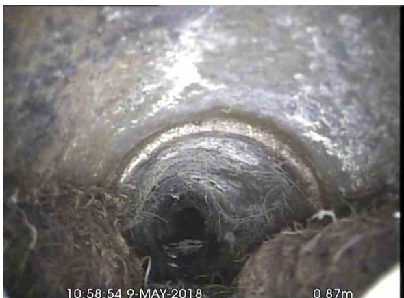
, 00:00:10, 0.87 m Roots, mass, 15% cross-sectional area loss, finish
