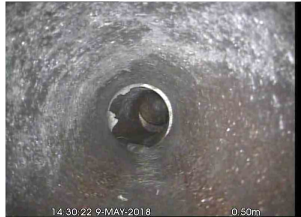
, 00:00:16, 0.50 m General photograph taken at this point
