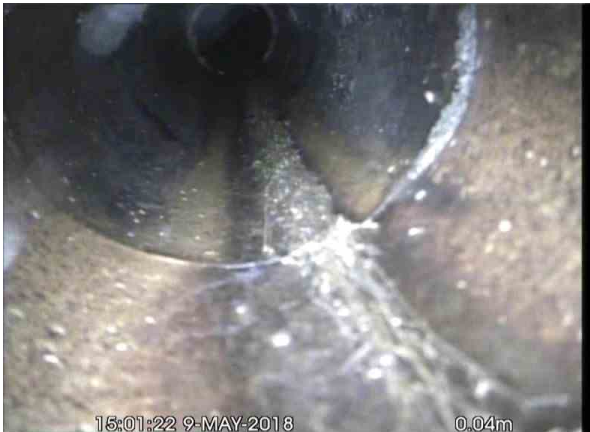
, 00:00:08, 0.04 m Roots, mass, 5% cross-sectional area loss, start
