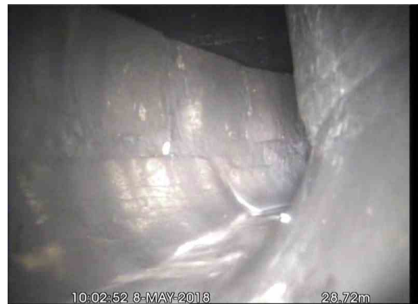
, 00:05:37, 28.72 m Finish node type, manhole, reference number: MH24 X
