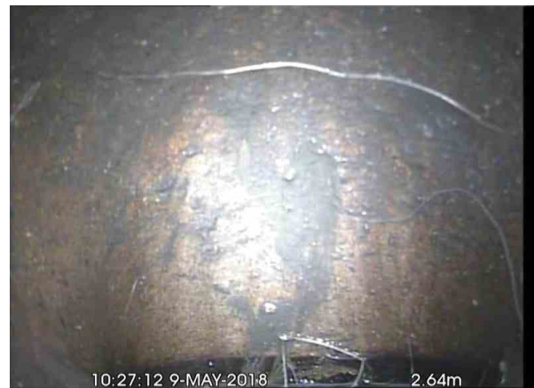
, 00:00:39, 2.64 m Finish node type, gully, reference number: Gully
