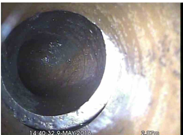
, 00:00:14, 2.07 m Material changes to vitrified clay
