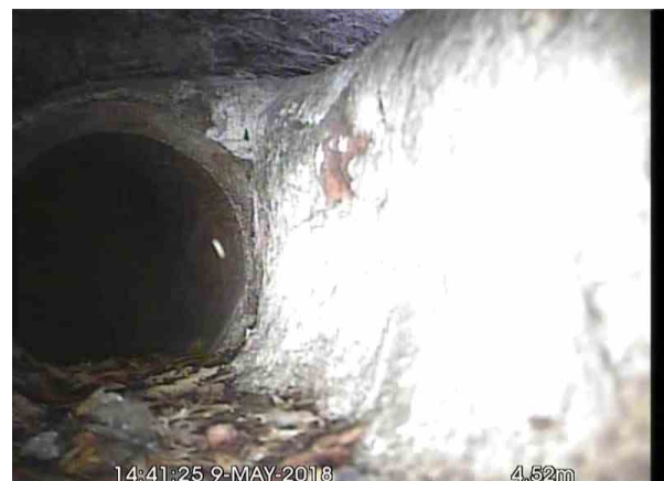
, 00:00:21, 4.52 m Finish node type, manhole, reference number: MH28 X
