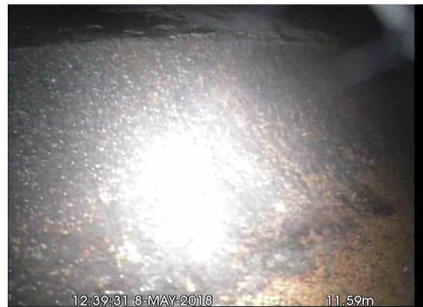
, 00:01:05, 11.59 m Finish node type, manhole, reference number: MH10 A
