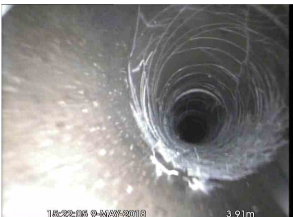
, 00:00:35, 3.91 m Roots, mass, 5% cross-sectional area loss, start
