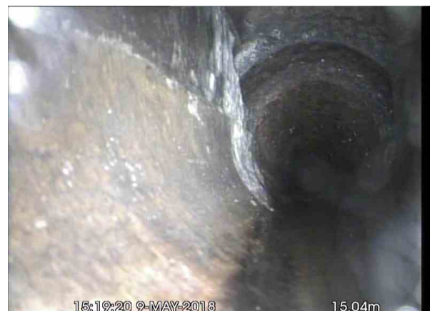
, 00:01:07, 15.04 m General remark, Camera passes through buried MH
